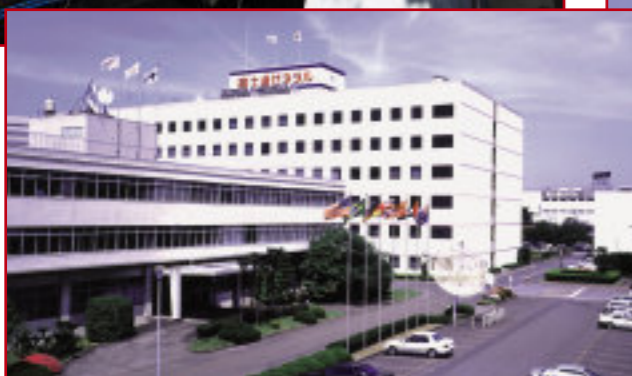
Headquarters Fujitsu General LTD (Japan)
